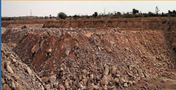
Continuous Backfilling
