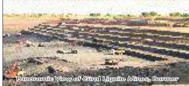
Panoramic View of Open Pit Lignite Mines, Barmer
