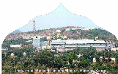
Industrial Beneficiation Plant, Jhama, Kota
